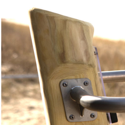
Construction made of Robinia - very durable acacia wood with a diameter of ~ 18 cm without sharp edges, resistant to weather conditions,
