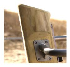
Construction made of Robinia - very durable acacia wood with a diameter of  $\sim 18$  cm without sharp edges, resistant to weather conditions,
